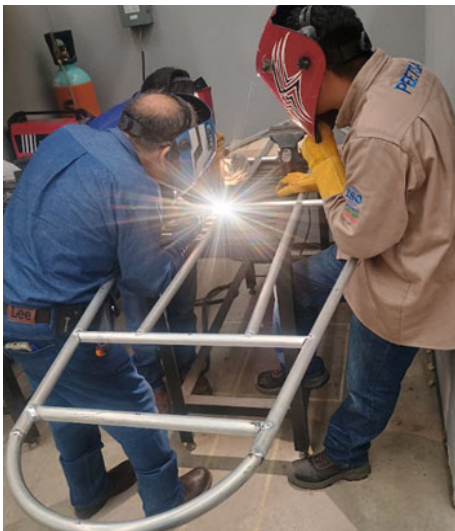
Fig. 15. TIG welding of the single-seater structure.
