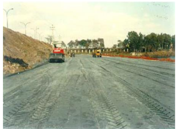
Figure 3: Nizamuddin Bridge Approach Road Embankment at New Delhi
