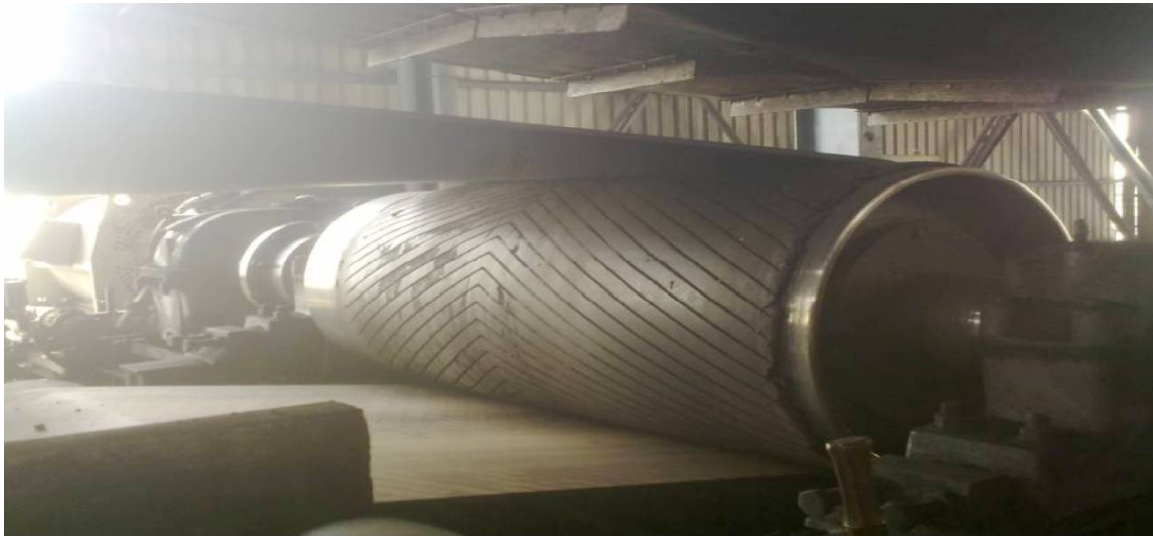
Figure 6: Installed Belt Cleaner at Driving Pulley
