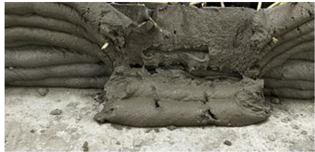
Figure 7. The phenomenon of structural failure is due to the material mixture not achieving plasticity.
