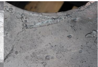
Figure 7. After blasting, cover plate surface
