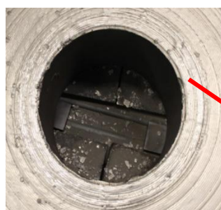
Figure 27. Re-Cladding of cover plate
