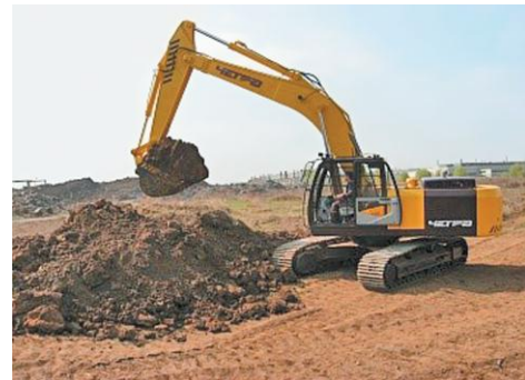
Figure 1. Single-bucket r excavator CHETRA EGP-230
