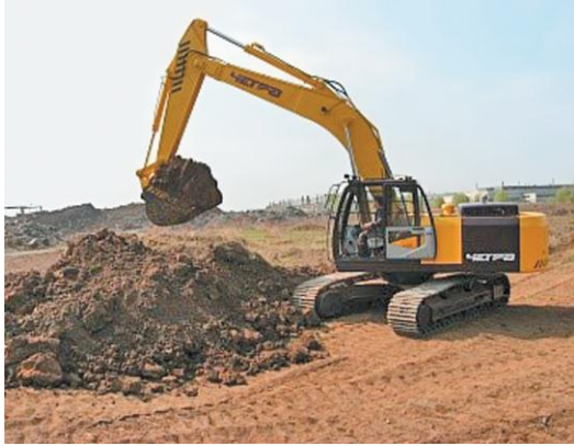
Figure 1. Crawler excavator CHETRA EGP-230
