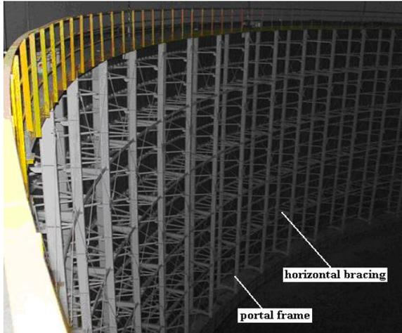
Figure 3. A new structural form of the piston retaining frame.
