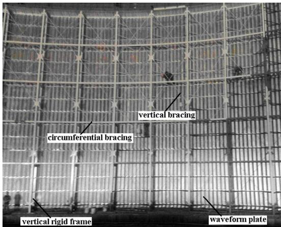
Figure 4. Partial of piston retaining frame.
