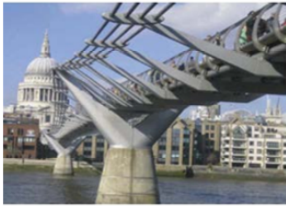
Figure 2: The London Millennium Bridge
