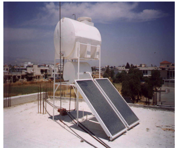
Figure 6: Thermosyphon Solar Water Heater
